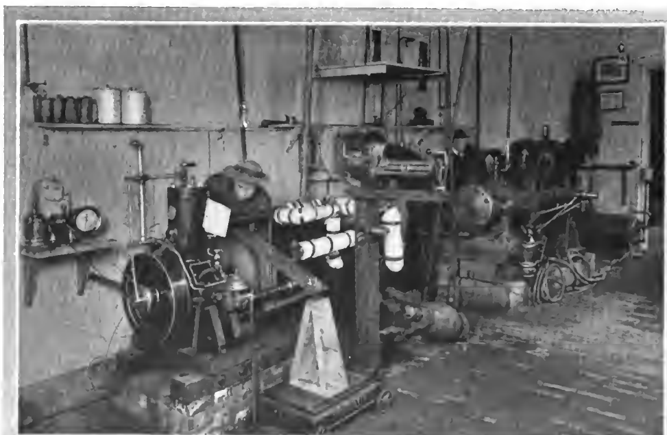
LOZIER MARINE ENGINE RIGGED FOR TESTING, IN SIBLEY COLLEGE LABORATORY.
